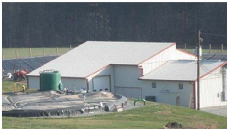
The community digester at Sensenig Dairy in Kirkwood, Pennsylvania is fed six times a day with manure from cows, hogs and chickens, and community food waste. The project has reduced emissions and operational costs, while creating additional revenue from the sale of carbon credits, fertilizer, and bedding.
